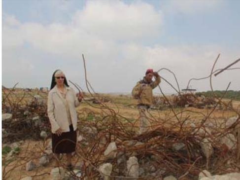
*These twisted steel rods will be straightened by a hand-operated machine and re-used.*
